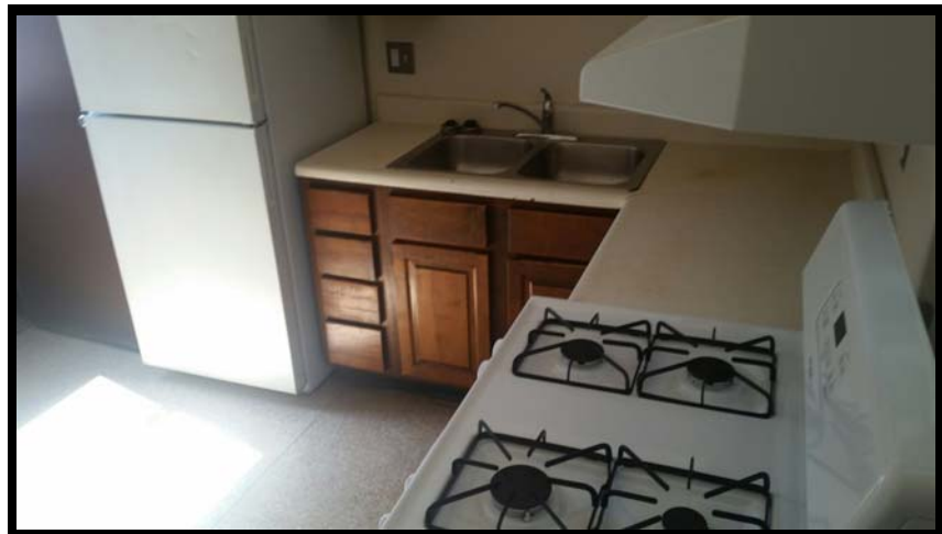
Typical kitchen (Desoto Bass Courts)
