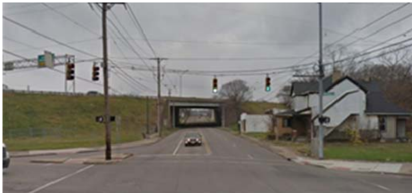
Existing – Germantown heading West at US35 overpass
