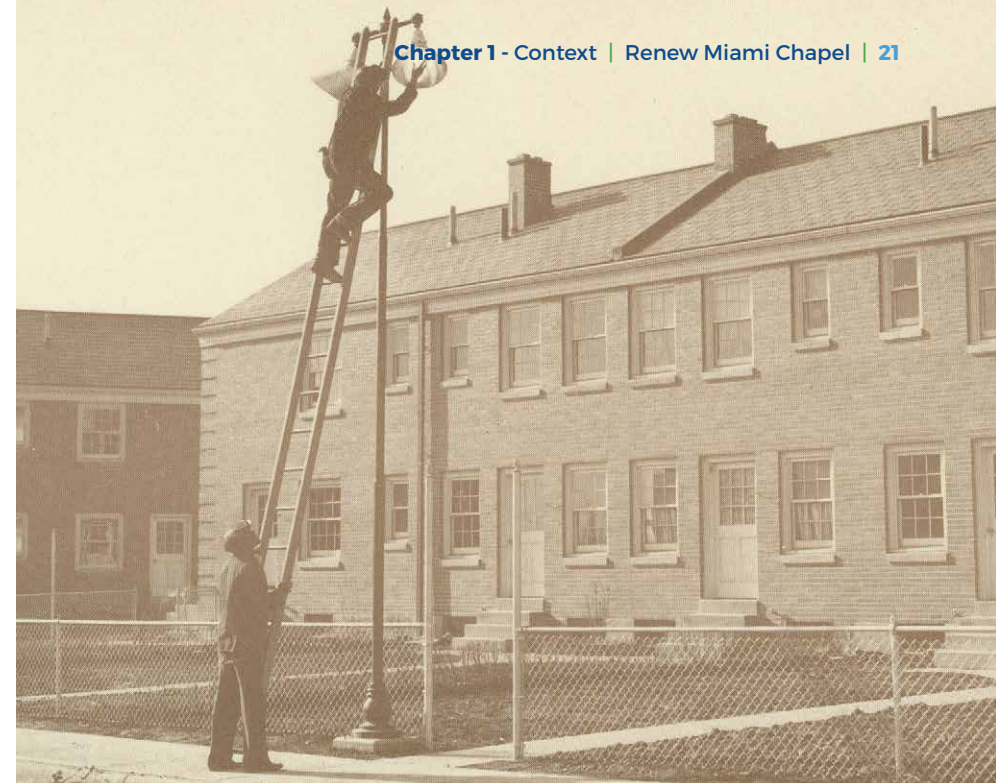
DeSoto Bass during construction, circa 1940.
